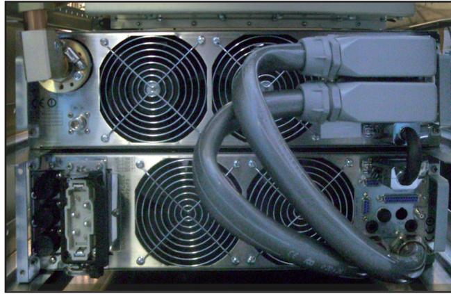
**Figure 5-1** Example of PJ4000/5000U-K installation in a rack
